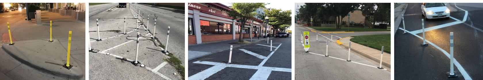
OmegaPost is a Category 1 small and light weight device with no attachments. Products such as these have been in common use for many years and are known to be crash worthy by testing of similar devices and years of demonstrable safe performance.
